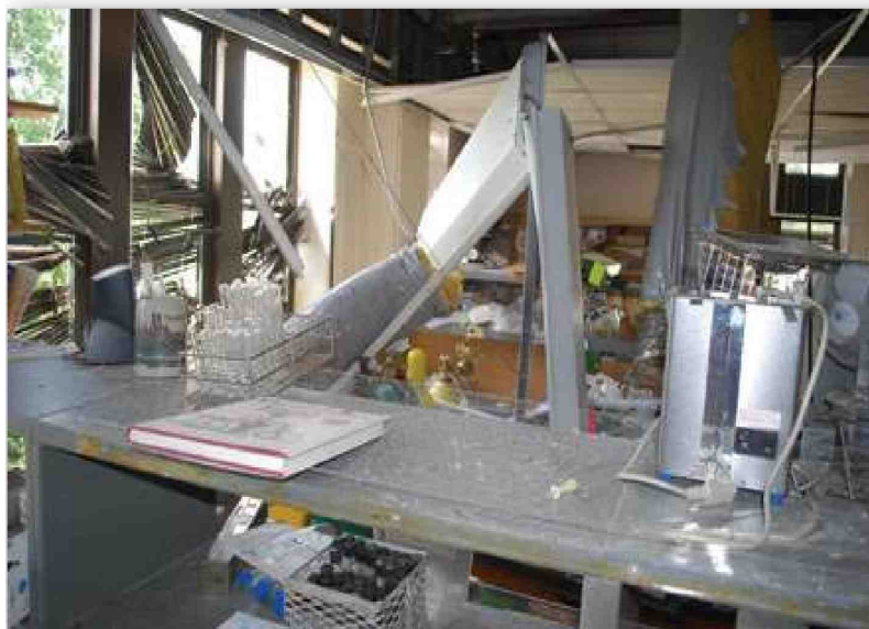
On June 28, 2010, an explosion caused by hydrogen gas in a University of Missouri biochemistry research lab injured four researchers and destroyed the laboratory.
